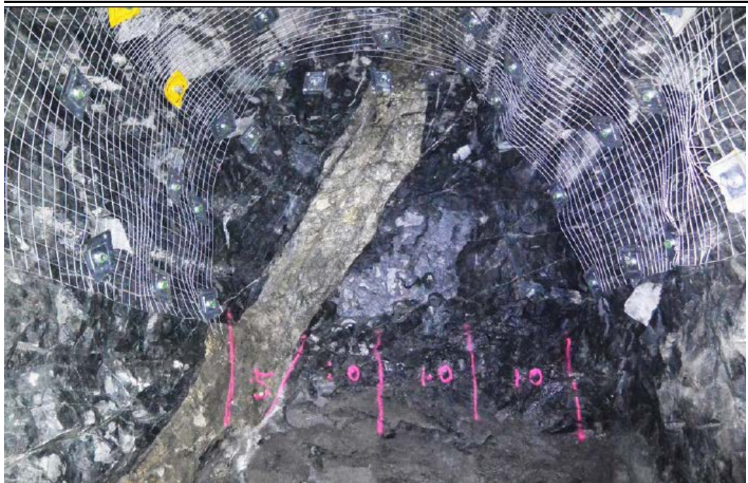
Figure 2: Link Lode as exposed in an ore drive
